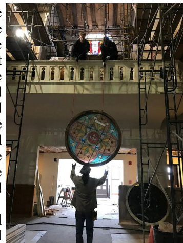
The windows being lowered from the Choir Loft
